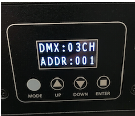
DMX CABLE CONNECTED
